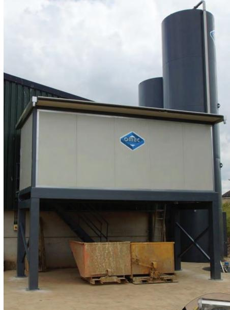
The OMEC system supplied by New Stone Age to Cumbrian Stone that can deliver 1,200 L/min of water, with back-up pumps throughout to ensure production continues if a pump fails.
