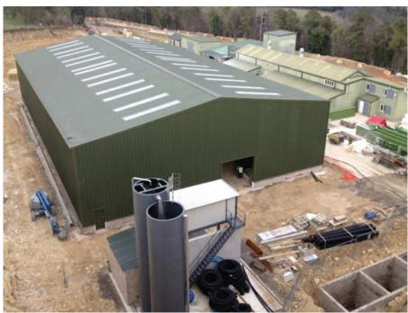
Meister Masonry's new factory in Painswick, Gloucestershire, with its OMEC water recycling system supplied by New Stone Age that will deliver 1,600 L/min of clean water.
